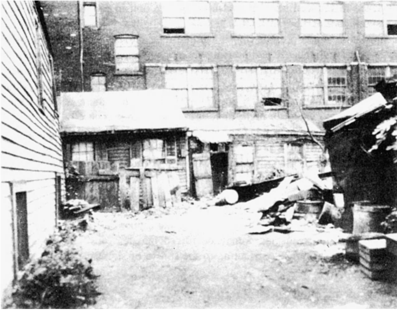
FIGURE 2.2 Run-down, filthy, vermin-infested backyards present many real health hazards.
