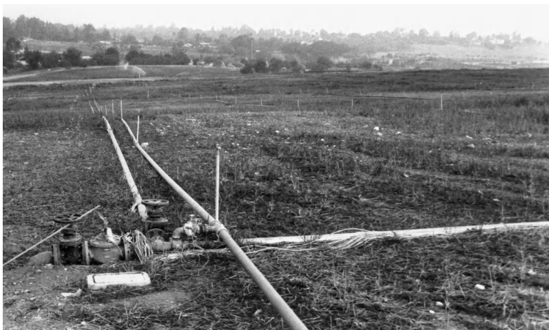
FIGURE 3.38 Completed landfill with irrigation system.
