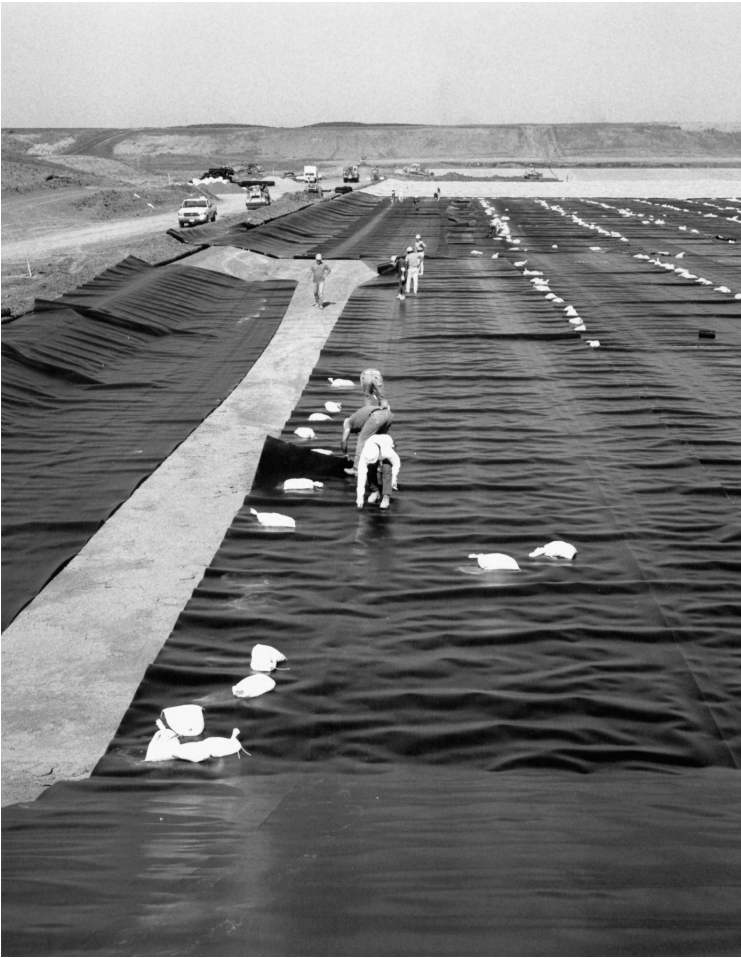
FIGURE 3.28 Placement of geomembrane liner in area-type landfill.
