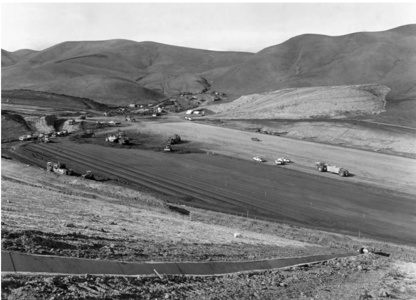
FIGURE 3.25 Development of large ravine landfill site. Equipment is compacting sub-base of landfill in preparation for placement of geomembrane liner.
